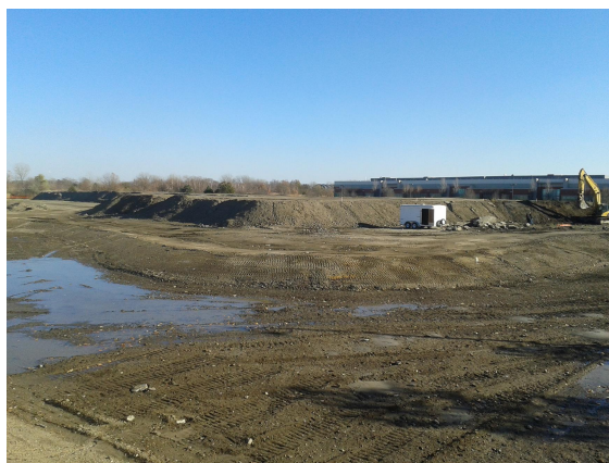
Overview of Surcharge Embankment
